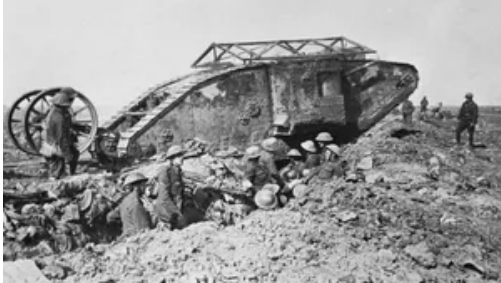
Mark I tank
